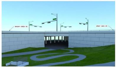
Artist rendering of side view when bridge is built. Hooded light signals atop the bridge ease access for turning vehicles while limiting any light pollution. Protected left turning lanes for all directions of the traffic.
