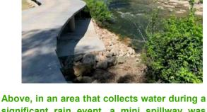
Above, in an area that collects water during a significant rain event, a mini spillway was built to direct that water into the creek. In the top picture, those rectangular slabs of concrete are where a water line is located.
