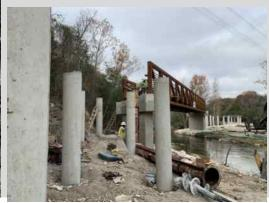
tly elevates to be level with the bridge (ADA compliant). Concrete columns have been placed for the boardwalk up to the bridge on both sides. In the far left, the beams have been placed on the columns. Sections of it are over a Round Rock wastewater line.
